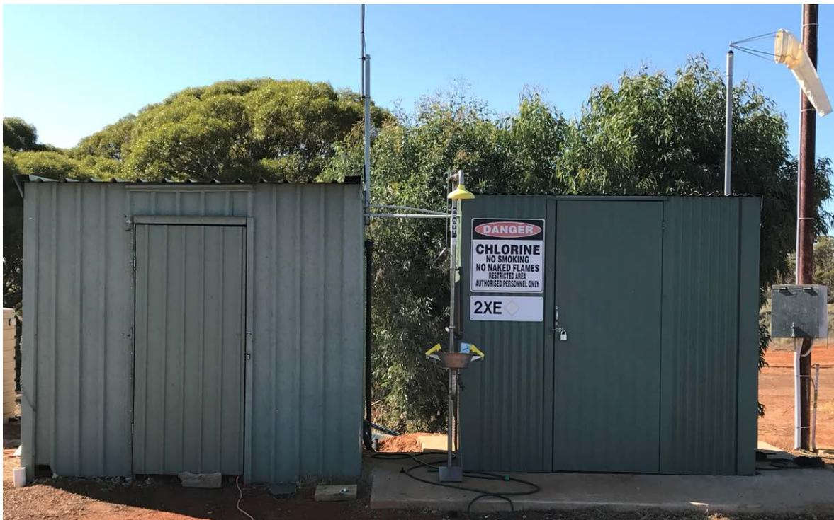
Chlorine gas is used to sanitise and achieve safe disinfection levels in the Shire wastewater reuse scheme. This method is approved by the Department of Health (DoH) has been used for many years. The use forms part of the licensing conditions and Recycled Water Quality Management Plan for the Shire of Yilgarn, endorsed by the DoH and the Department of Environment and Water Regulation DEWR.
