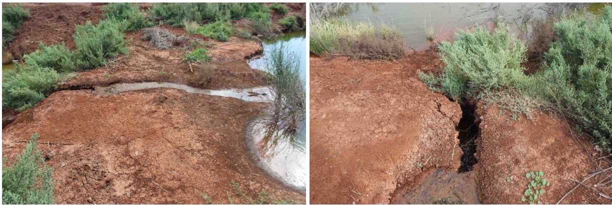
Figure 11: Erosion between primary and secondary ponds
