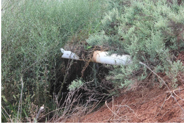
Figure 10: Broken interconnecting pipe between primary and secondary ponds
