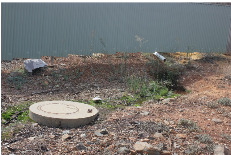
Figure 5: Overflow from camp water tank eroding around AC1B13
