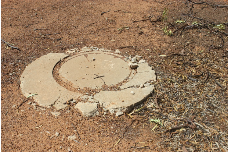
Figure 3: Access Chamber AC1A5 needs replacing
