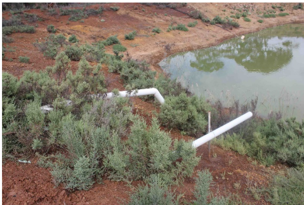
Figure 12: Blocked pipes between secondary and tertiary ponds
