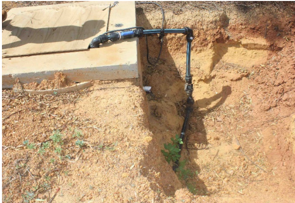
Figure 9: Temporary pressure main bypass at PW002 (PS2)
