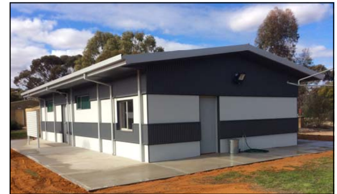
New upgraded ablution block
