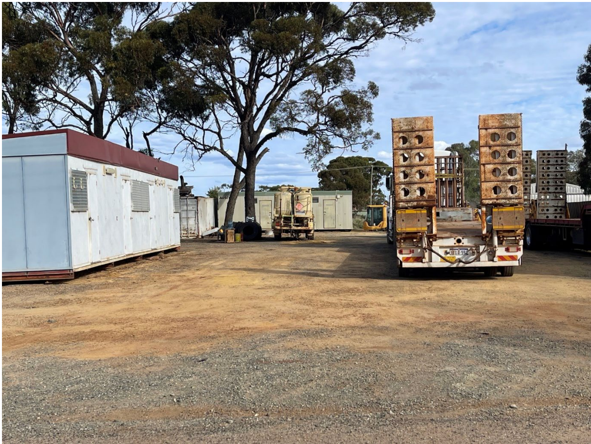
Figure 5 - Close up of transportable buildings located at rear of subject site
