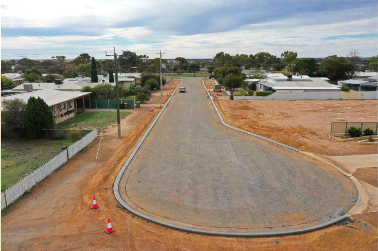
Completed kerbing on Libra Place
