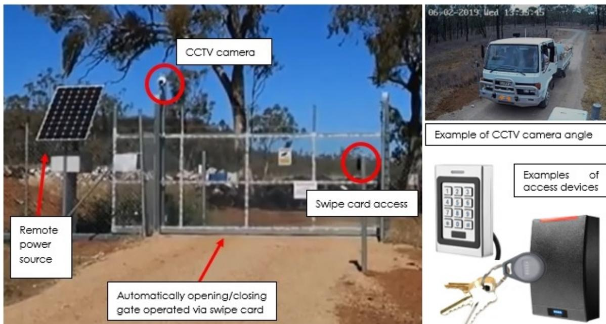
This system can be used for both landfills and transfer stations and has the added benefit of recording data about who is using the facility, at what time, and how often.
