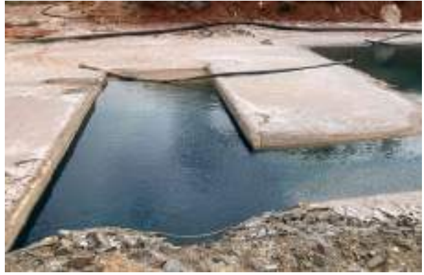
Photograph 3.4 Pump sump and sediment deposition at upstream end (left) and concrete sump (right)
