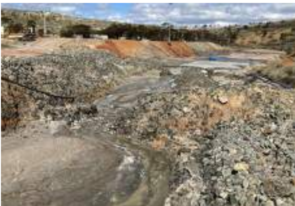
Photograph 3.3 Condition of drain below culverts and flowing towards toe pump sump. Looking downstream (left) and upstream from pump sump (right)
