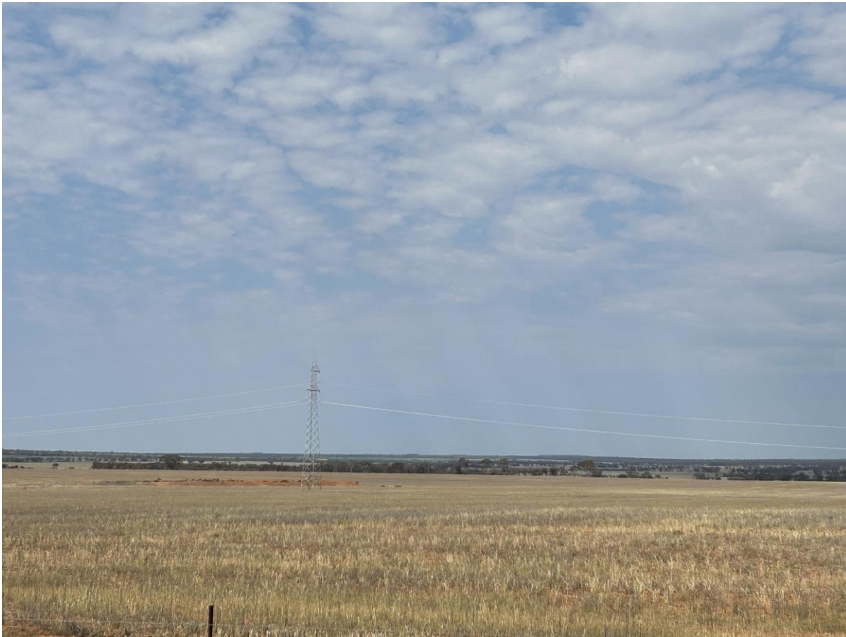
Figure 8 Transmission line located in central Project Area
