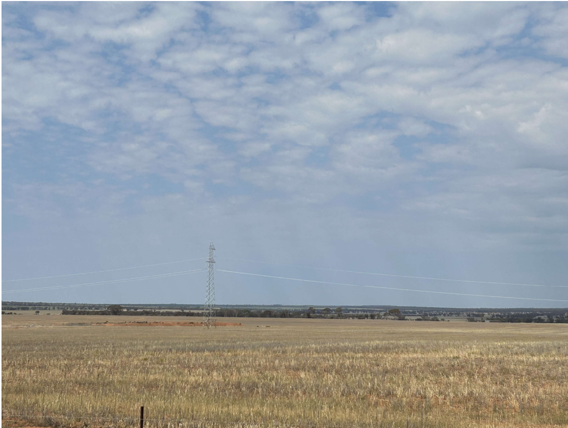
Figure 8 Transmission line located in central Project Area
